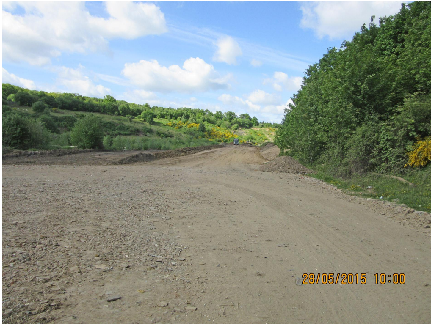
Figure 4 : View of haul road construction on 28 May 2015, facing southwest
